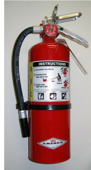
Fig. 4-2 - A good multi-purpose fire extinguisher for A, B, and C fires (dry chemical based).
