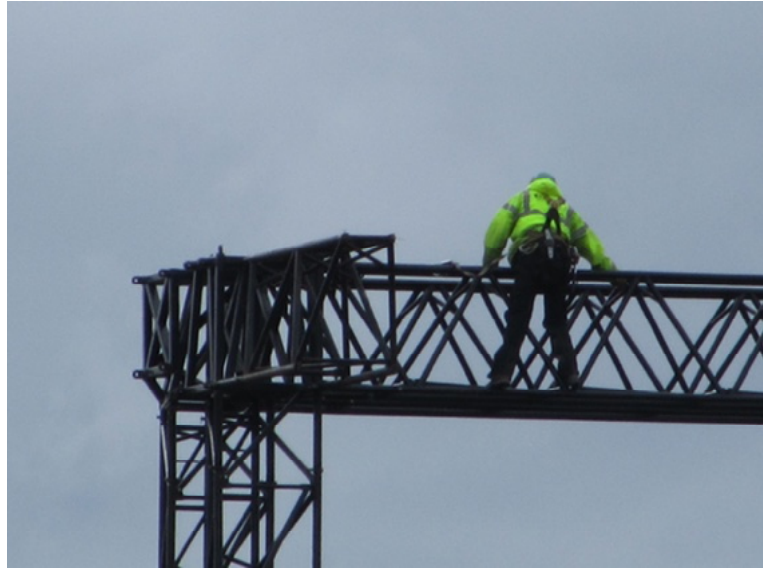
Fig. 19-2 – Example of a climber clipped in on a wet day. This is an example of appropriate fall protection. Photo courtesy of The Event Safety Shop, LTD.
