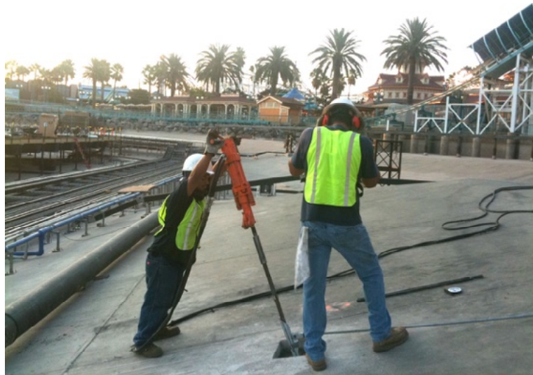
Fig. 19-1 – Installing an Earth Anchor. Earth anchors can be an effective and space efficient alternative to using bulk weight to ballast structures and rigging.
