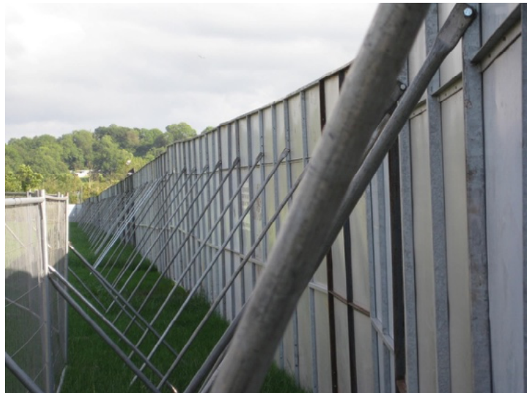
Fig. 23-4 - Solid temporary fence panels showing diagonal bracing. This is a pedestrian barrier used to channel queue lanes – perfect when no sideways pressure is anticipated. Photo courtesy of The Event Safety Shop, LTD.
