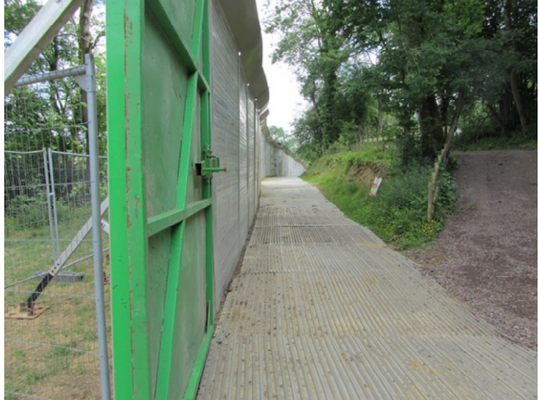
Fig. 23-5 - A custom-made fence designed to create an impregnable event perimeter. Block and mesh panels form an inner fence to create a moat in which security can operate.. Photo courtesy of The Event Safety Shop, LTD.
