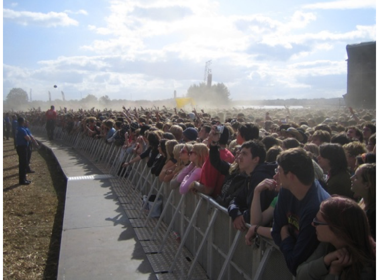
Fig. 23-6 - A standard concert stage barrier, note the diagonal bracing stays which allow the barrier to resist horizontal load. Note also the extended rear plate allowing security personnel easy access and a safe platform from which to assist or rescue the public. Photo courtesy of The Event Safety Shop, LTD.
